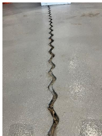
Anti hit deformation joint
